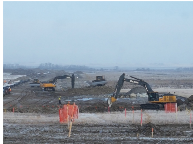
16. Bore pits being covered – km 161+000 – Jan 26, 2018
