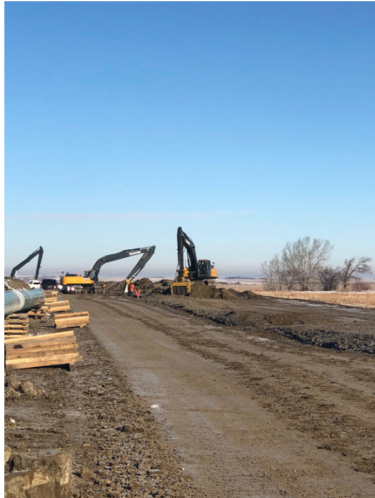
1. Backfill tie-in– km 168+530 – Jan 23, 2018
