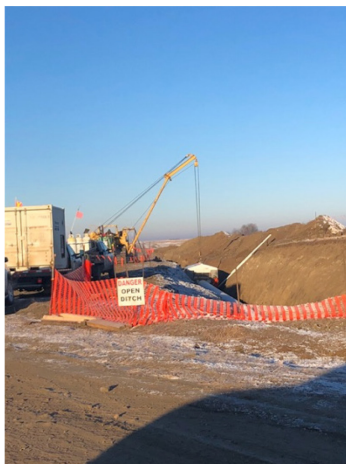
5. Tie-in weld – Km 163+370 – Jan 23, 2018
