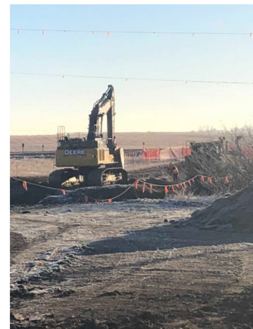
6. Excavator and dozer – Km 163+550 – Jan 23, 2018
