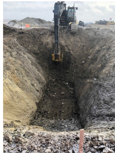
18. Slip bore digging catch pit - km168+950 – Jan 26, 2018
