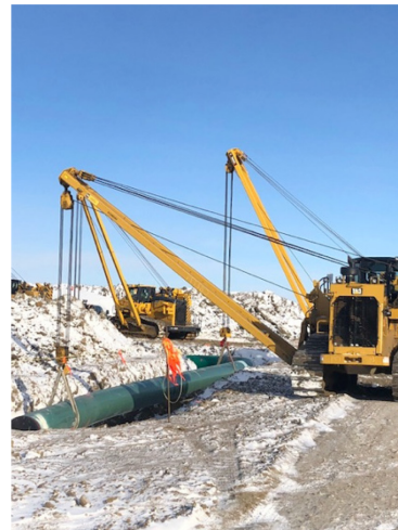
22. Booms on tie-in - km 169+500 – Jan 27, 2018
