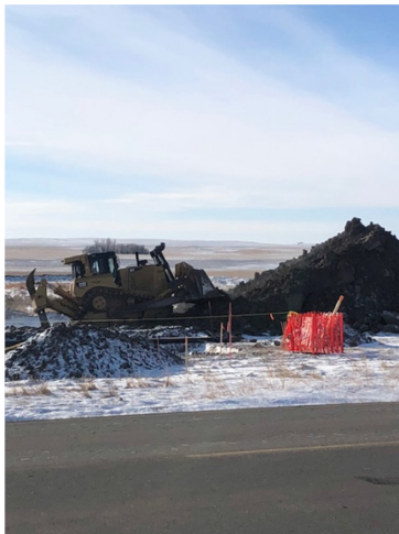
21. Dozer pushing dirt – km 166+450 – Jan 27, 2018
