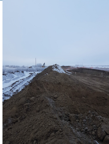
8. Spill pile - Km 163+550 – Jan 24, 2018
