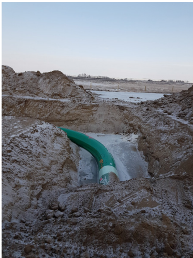
17. Uncovered bend -160+450 - Jan 26, 2018
