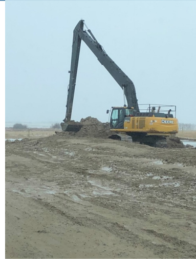
20. Excavator dig - km160+467 – Jan 26, 2018
