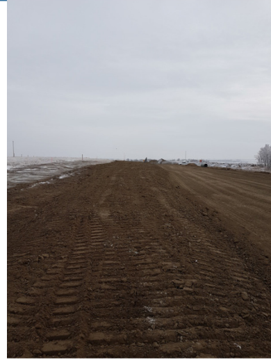
14. Tie-in Backfill- Km 163+300 – Jan 25, 2018
