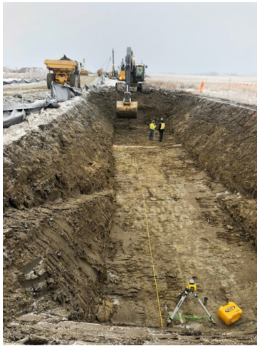
9. Bore pit - km 166 (SF 98)– Jan 24, 2018
