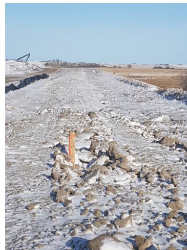
24. Tie-in backfill – Km 160+900 – Jan 27, 2018
