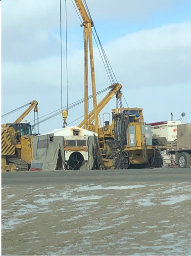
19. Booms on bore crew- km166+450 – Jan 26, 2018
