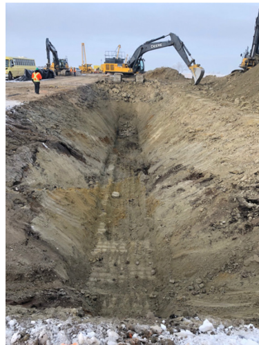
12. Bore bay – km 162+910 – Jan 25, 2018
