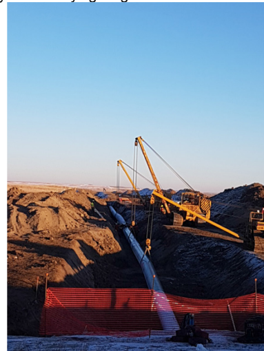
4. Tie-in - Km 159+450 – Jan 23, 2018
