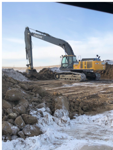
23. Excavator digging in soils for spring run-off – km 159+600 – Jan 27, 2018
