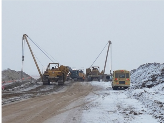
7. Tie-in – Km 160+300 – Jan 24, 2018
