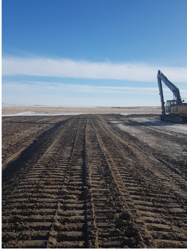
25. Tie-in Backfill – km 160+400 – Jan 27, 2018
