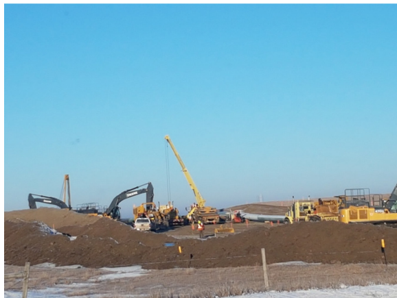
3. Unloading pipes - km159+450 – Jan 23, 2018
